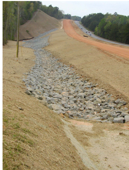
Large rocks for channel reinforcement and to reduce the velocity.
