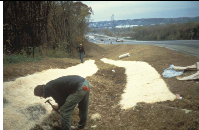
Installation of reinforced liner along thalweg of channel, with other material along sides (VA photo).
