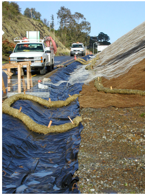
Plastic tarp, with coir logs, for a temporary liner and to slow the velocity.
